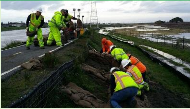
SCVWD EA Crew on the levee, building "chimneys" with sandbags.
